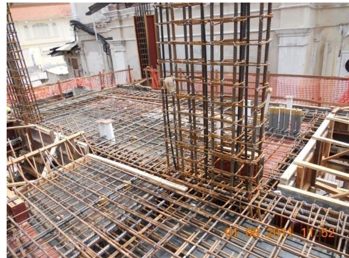
Re-bar checking and casting of slab @ 1 st storey Slab @ grid line 6A-10C
