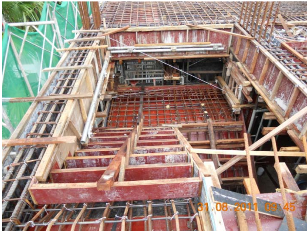
re-bar , formwork checking before casting of last portion of Grid Line 1A-6A 2 nd storey slab
