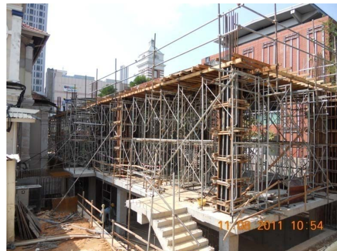
erection of staging from grid line A1-10C for 2 nd storey slab
