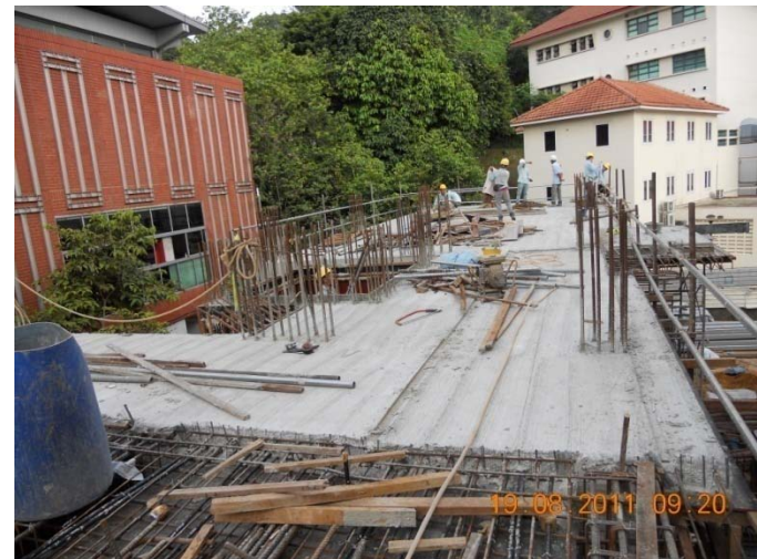
Re-bar Checking before casting of 2 nd storey slab and after casting
