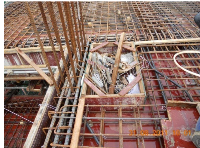
re-bar , formwork checking before casting of last portion of Grid Line 1A-6A 2 nd storey slab
