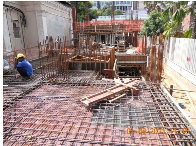
staging, formwork, re-bar of Slab @ Grid 6A-10C
