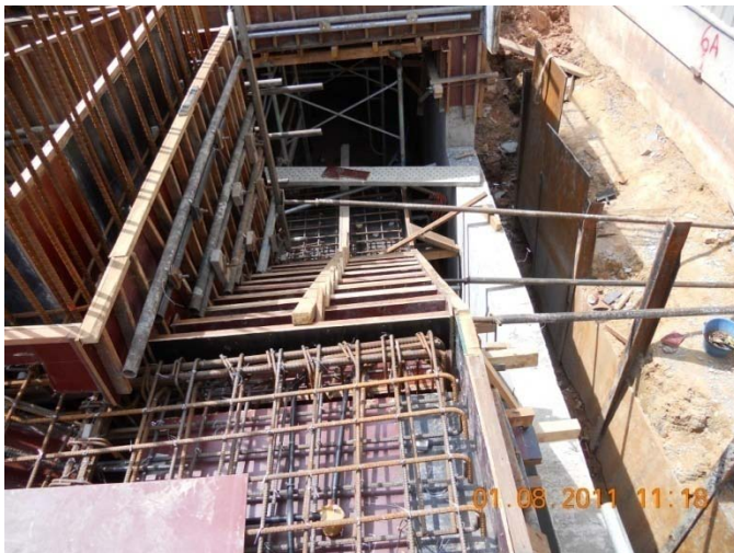
Re-bar checking and casting of slab @ 1 st storey Slab @ grid line 6A-10C
