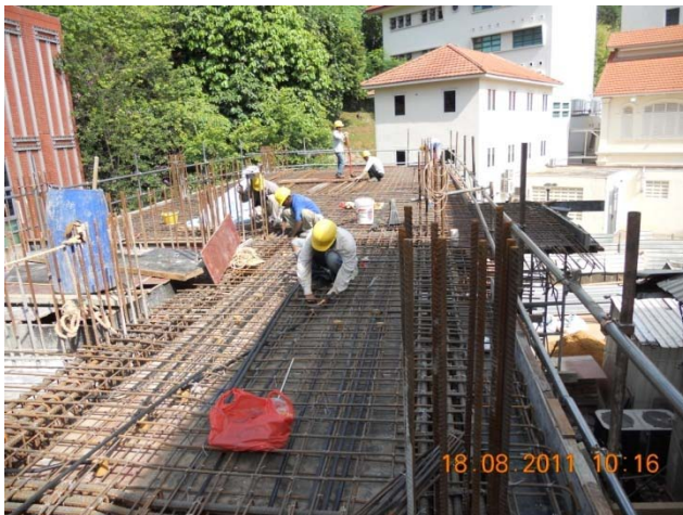
Re-bar Checking before casting of 2 nd storey slab and after casting
