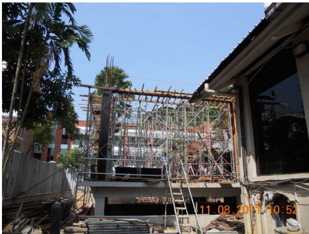
erection of staging from grid line A1-10C for 2 nd storey slab
